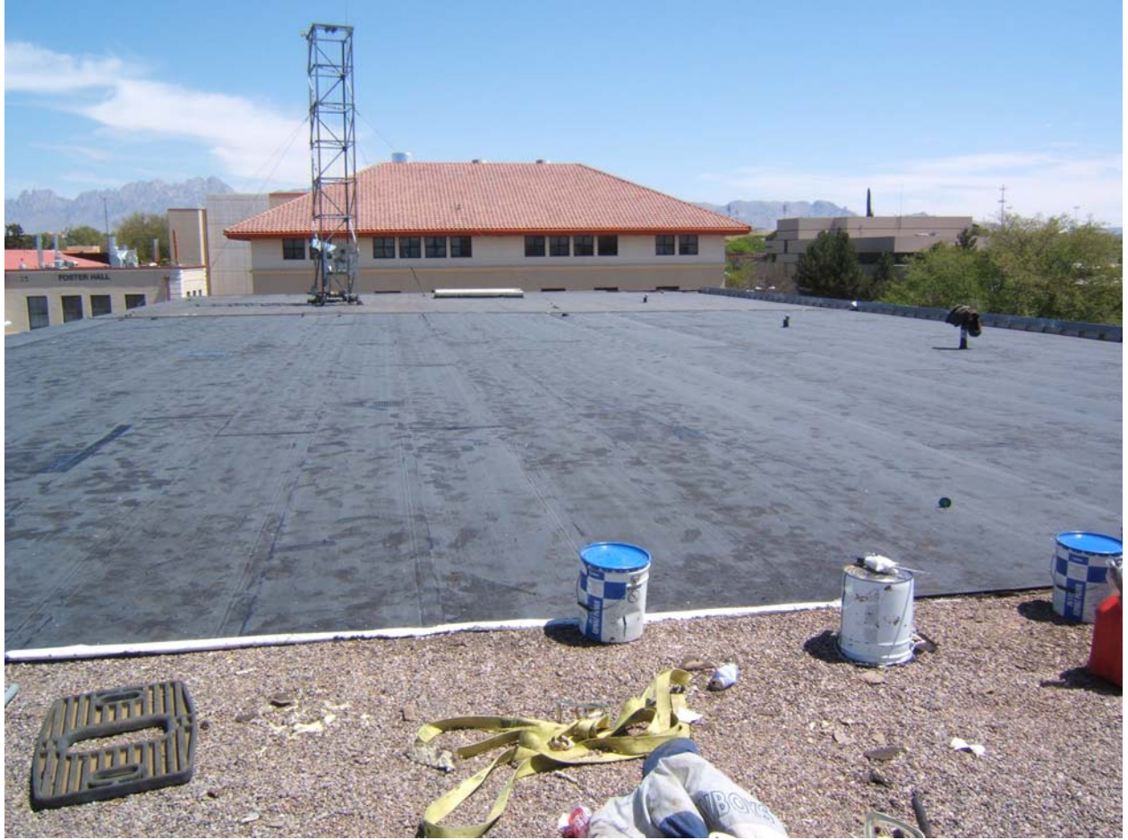
Figure 3 - Placing new tar paper on the surface.
