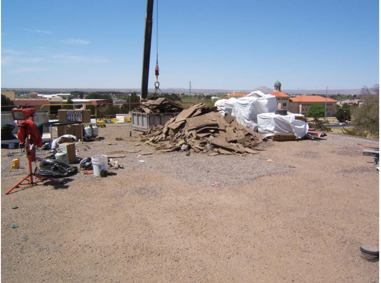
Figure 2 - Hauling down old materials by crane.
