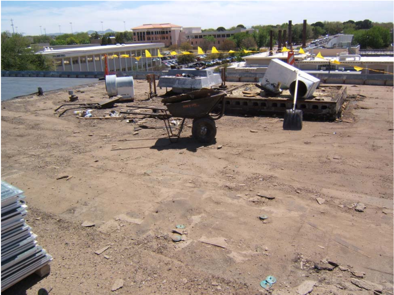
Figure 1 - Scraping off the old stones and surface materials
